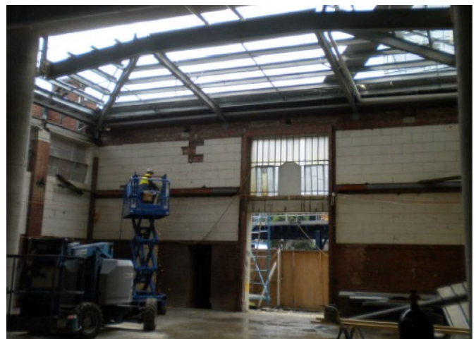
Main Hall during renovation. Source: Housing Choices Australia
