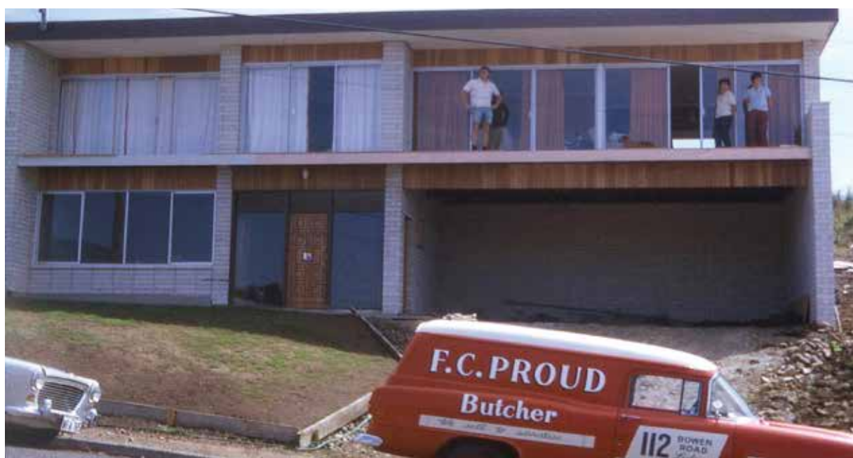
New home build Hobart, 1969 – low energy efficiency, non-universal design
