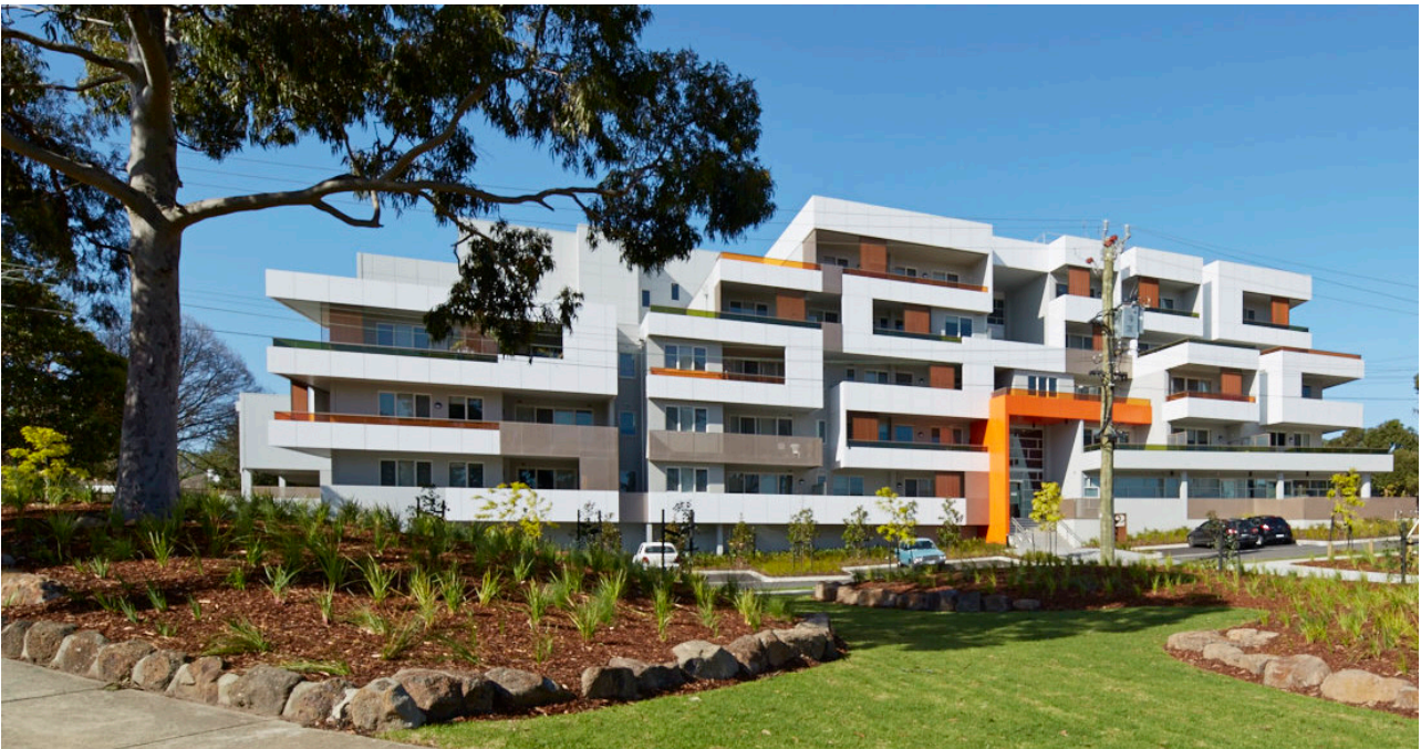
Ashwood Chadstone Gateway exterior
