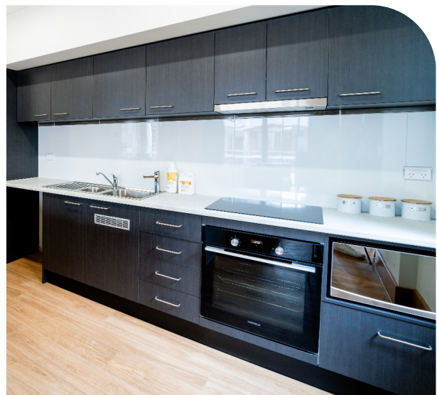
The light-filled kitchens are modern and allow for very easy maintenance
