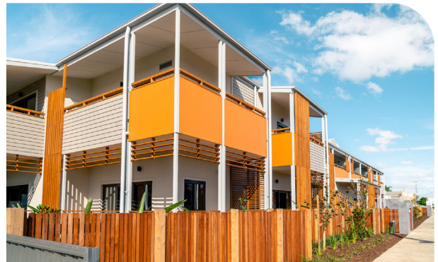
Jimmy Kennedy social housing units – exterior
